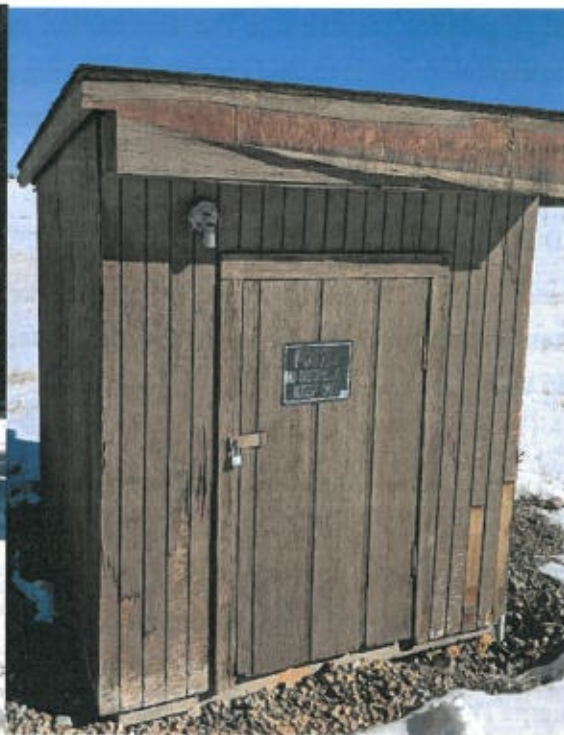
Figure 4: Control Building B
